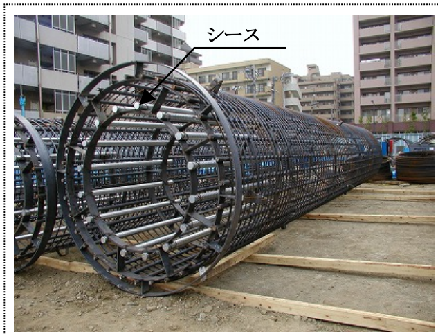
写真-2 杭の鉄筋かごの組立て
